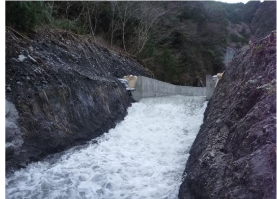
[地山掘割水路部]
