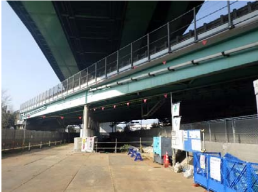
吊り足場架設前
