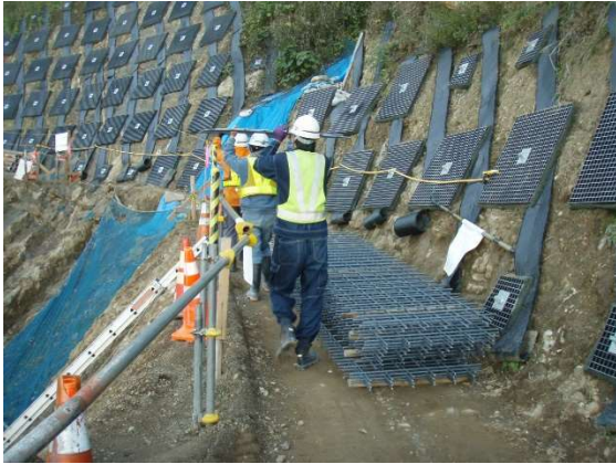
(資材運搬状況)
