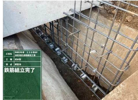
[鉄筋組立完了時]
