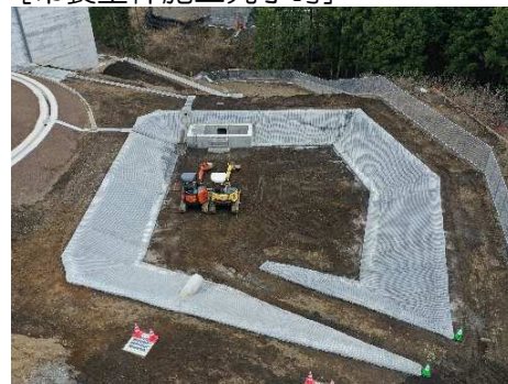
[布製型枠施工完了時]
